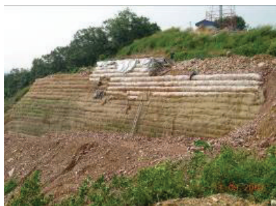
Figure 4. Wrap around reinforcement facing with coconut fibre ECM.
