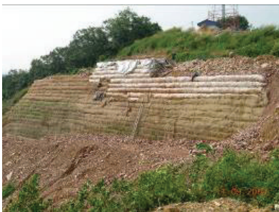
Figure 4. Wrap around reinforcement facing with coconut fibre ECM.
