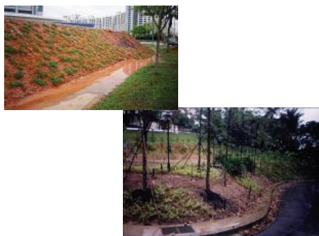
Figure 1. Examples of urban road side construction with serious erosion and sediment concerns
