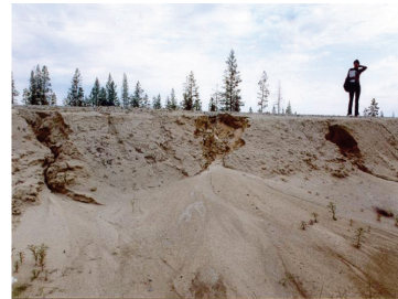
Figure 5. General view of unprotected slope section of Tarco Sale-Pionerny road.
