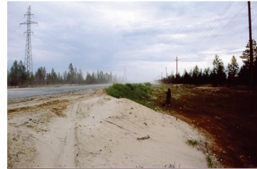
Figure 4. General view of adjacent sections of protected and unprotected slopes.
