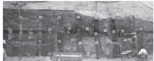
Photograph 3. Photo of actual application of geogrid slope surface protection.
