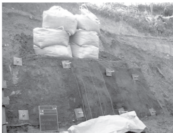
Photograph 1. Surcharge by soil pack.
