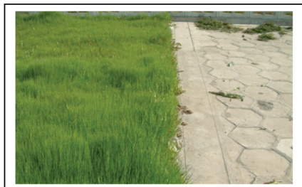
Figure 2. The comparison between ecological lawn slope protection and the concrete slope protection.
