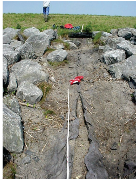
Figure 3. Photograph of broken sewn seams (stones removed).
