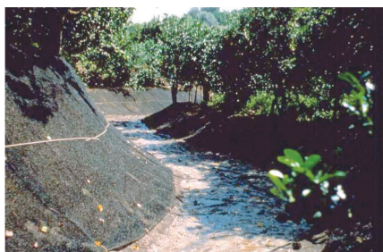
Figure 9. At the end of construction.
