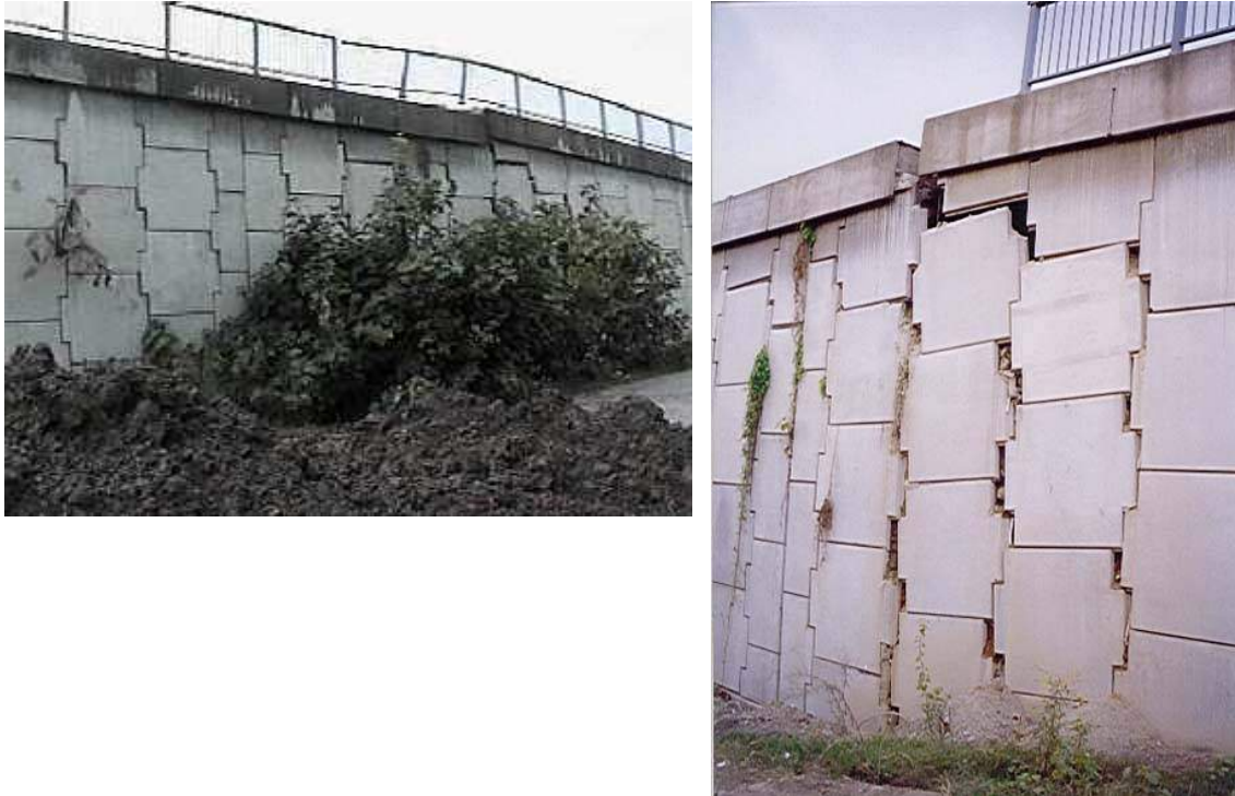
Figure 7. Reinforced Earth wall damaged in the Kocaeli Earthquake prior to demolition.
