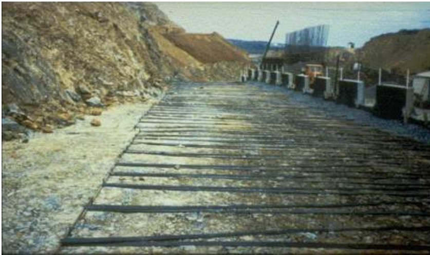
Figure 5. Wall under construction with 'Greywacke' cut face on left and reinforcement elements laid out.
