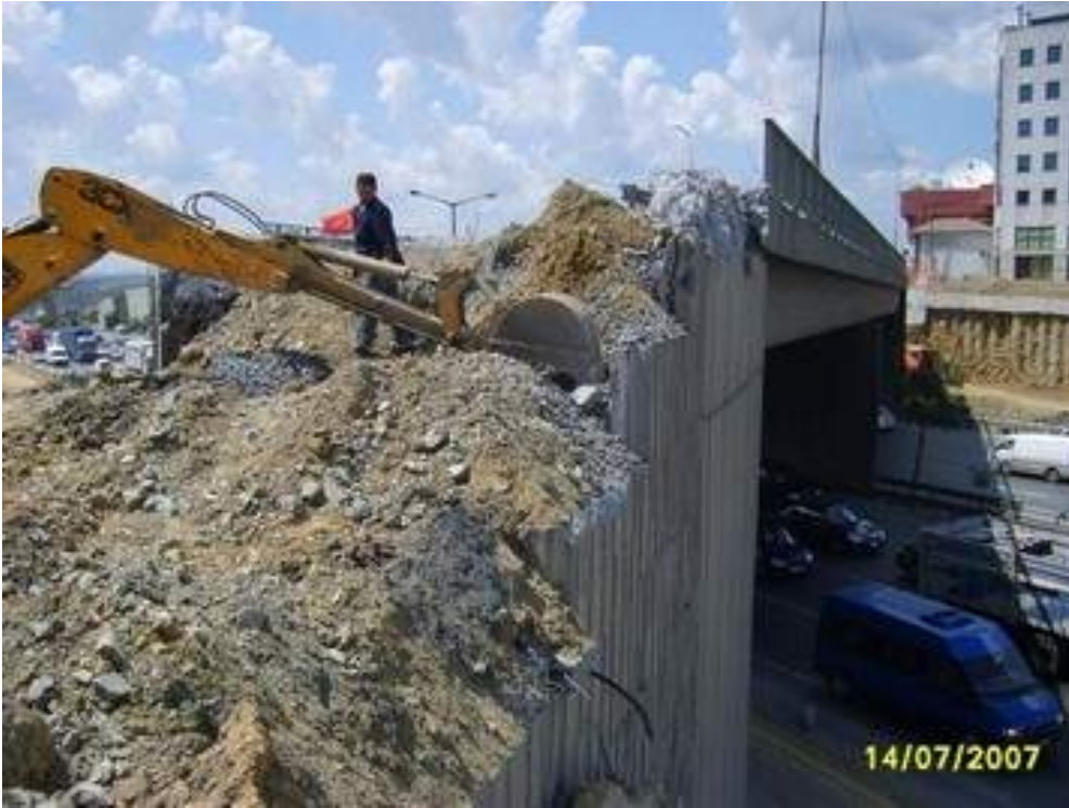
Figure 8. Demolition of the polymeric reinforced soil wall.
