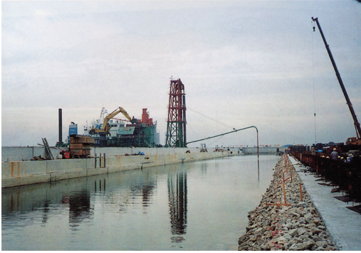
Photo 1. A working vessel placing lightweight soil underwater behind port structure.
