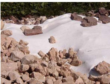
Figure 3. Gravel layer for base drainage with sharp corners
