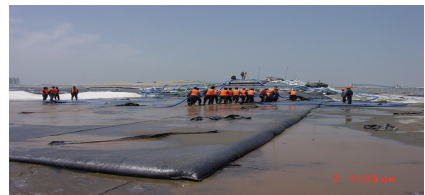
Photo 1. Panorama of the filled flat geotube embankment in practical engineering
