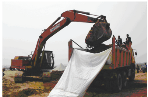
Figure 6. Mechanical cast loose soils.
