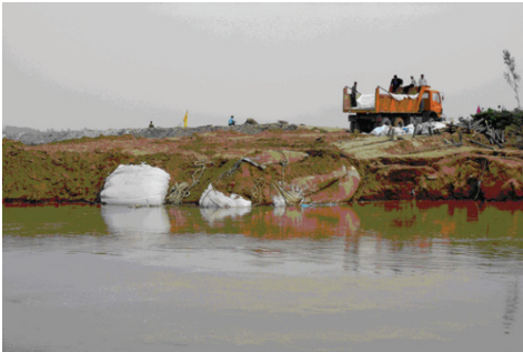
Figure 7. Underwater execution of large geocontainer.
