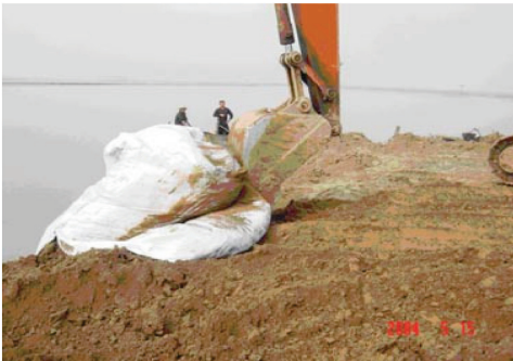
Figure 2. Geocontainer pushed by digging mechanics.
