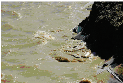
Figure 8. Resisting current scour of large geocontainer.
