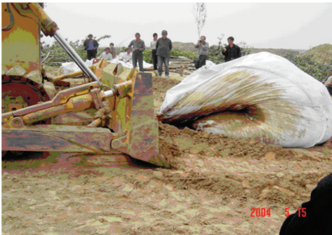
Figure 1. Geocontainer pushed by bulldozer.
