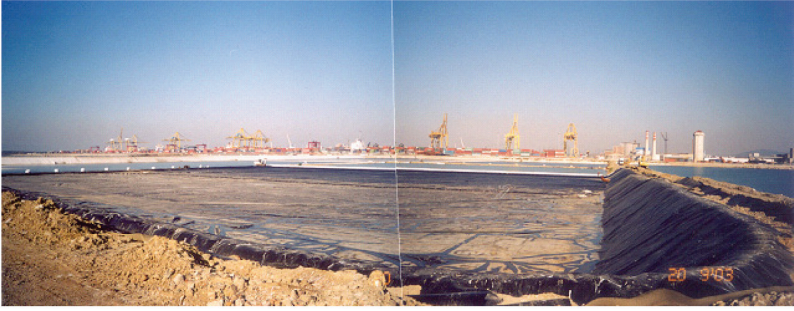
Figure 1. HDPE liner installed in an Italian harbour.
