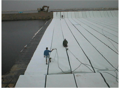
Figure 3. HDPE geomembranes pre-coated with geotextile. Geocomposites are 2 m wide (supplier contractor Macko).
