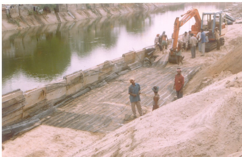
Figure 6. The wall under construction
