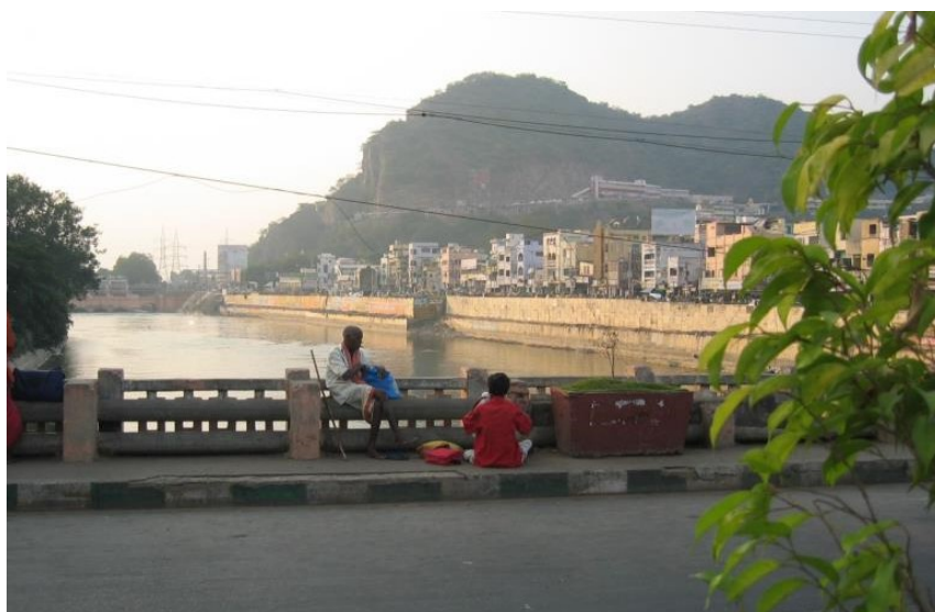
Figure 7. A view of the completed wall adjoining the canal
