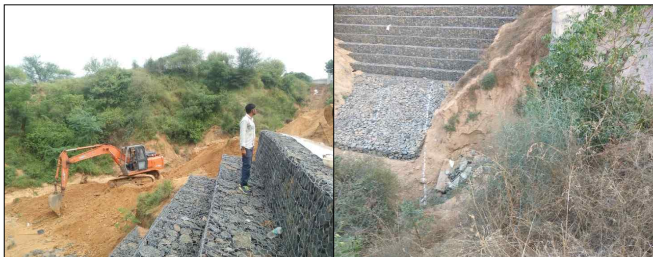
Figure 7: Gabion gravity with gabion mattress after construction
