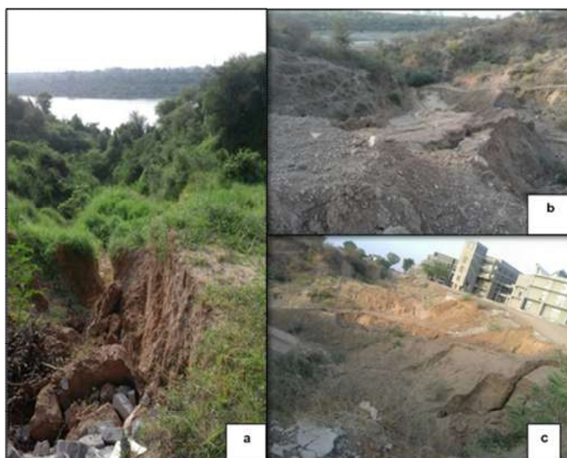
Figure 1: Eroded ravines in the campus along the bank of Sabarmati river
