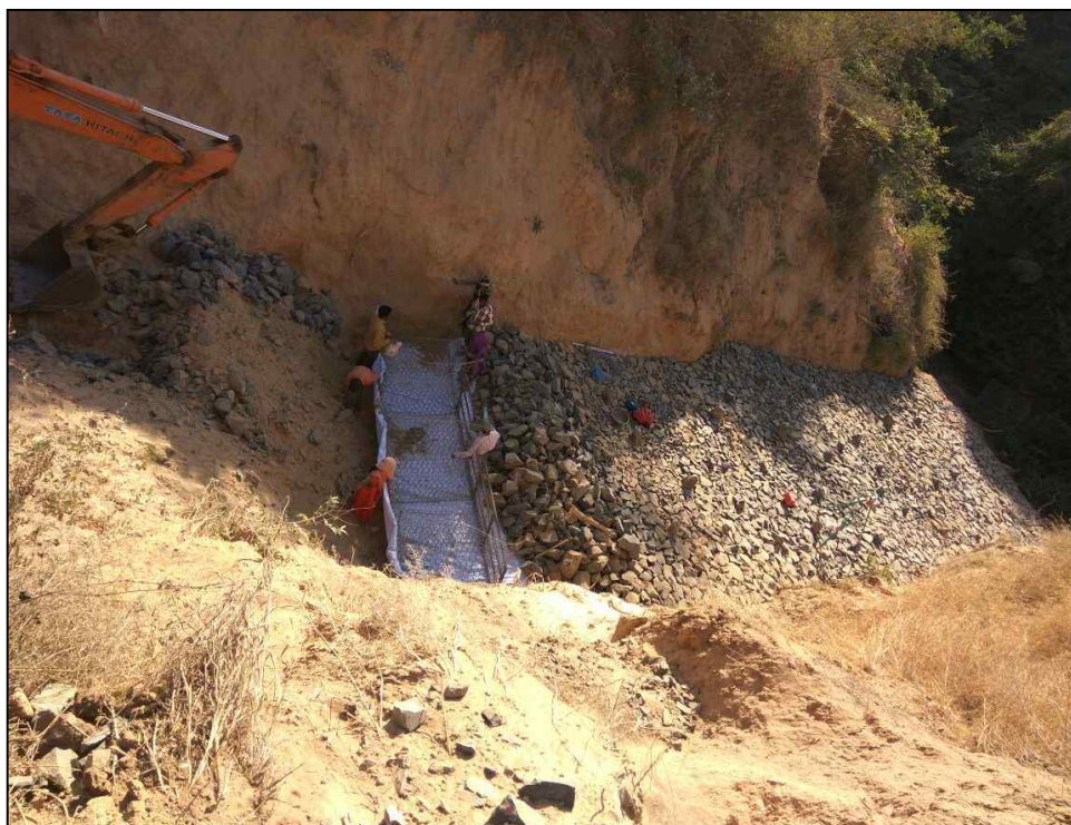
Figure 5: Placing non-woven geotextile between retained fill material and gabion box
