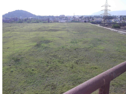
Capped Surface, Vegetated with irrigation system to maintain greenery
