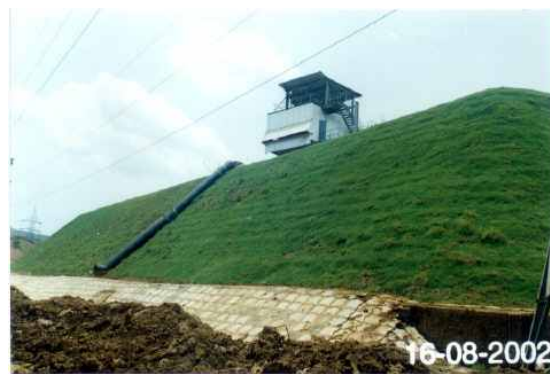
Perforated Pipe and Main connected to pumping system
