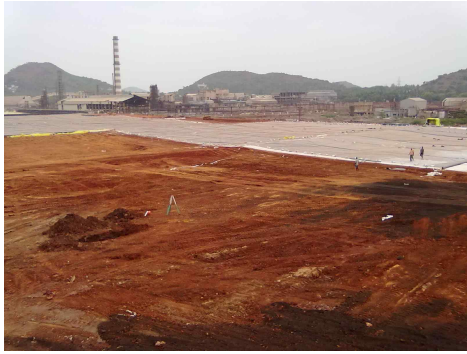
Strengthened surface and HDPE Liner Liad
