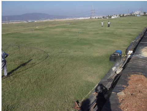
Capped Surface, Vegetated with irrigation system to maintain greenery
