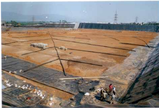
Perforated Pipe and Main connected to pumping system
