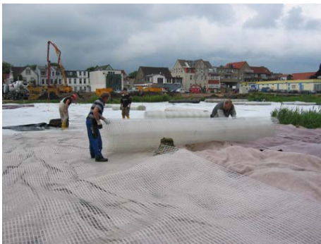
Photograph 5. Installation of Secugrid 200/40 R6 above Secutex R 504
