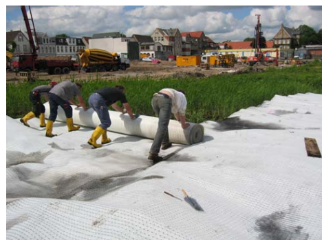
Photograph 4. Installation of Combigrid 60/60 Q6 (polyester) R 156
