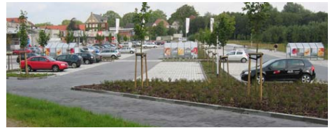
Photograph 9. Finished parking area
