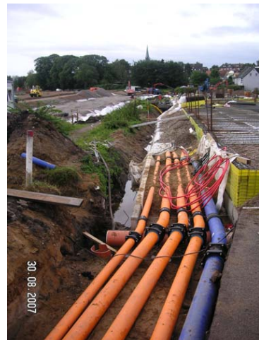
Photograph 2. Re-installation of the service pipes
