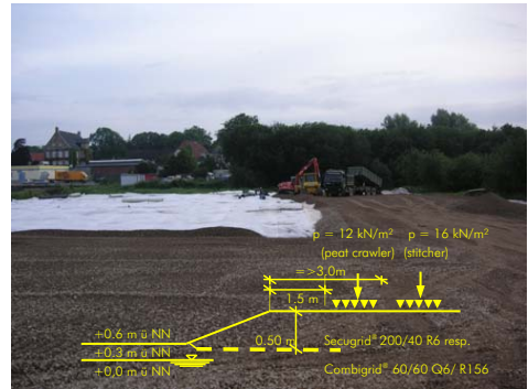
Photograph 6. Installation of the first filling
