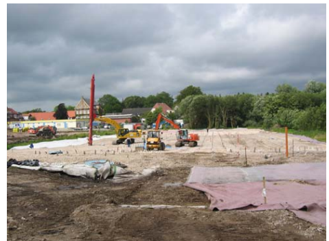
Photograph 7. Installation of the vertical drains
