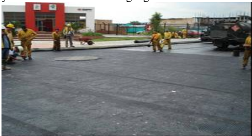
Picture 3. Roadwork after fiberglass application
