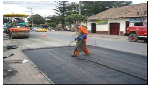
Picture 1. Roadwork after fiberglass application.
