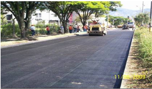
Picture 2. Roadwork after fiberglass application
