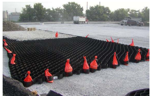
Figure 1. Geocell reinforcement road and subgrade applications
