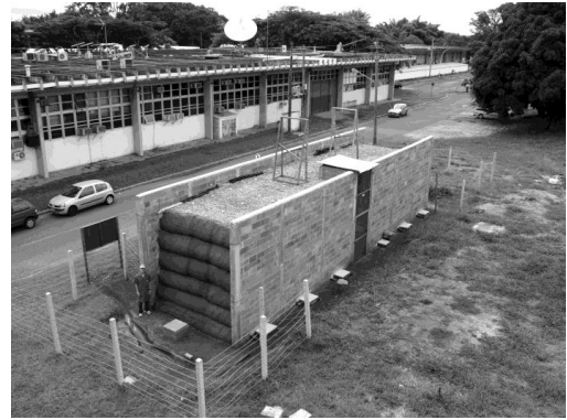
Figure 2. Reinforced wall test facility.
