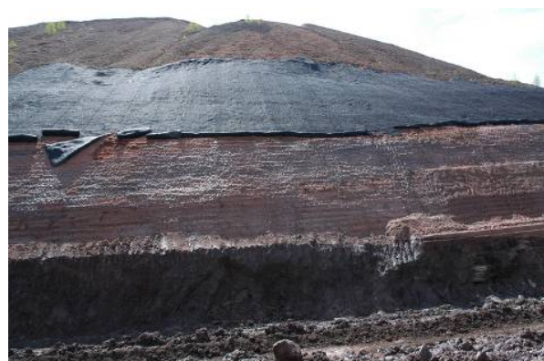
Figure 19...20: Erosion protection on a potash tailings pile (during construction)
