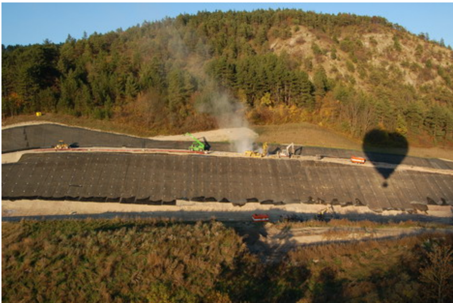
Figure 15: The slope under construction / placing the erosion protection mat
