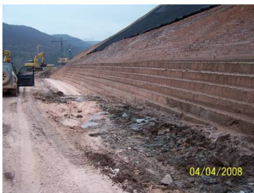
Figure 19...20: Erosion protection on a potash tailings pile (during construction)
