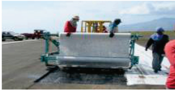
Figure 5. Installation of paving fabric with a mechanical rig.
