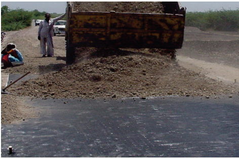
Figure 4. View of the road during laying of geotextile.
