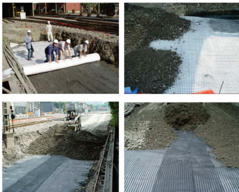
Figure 5. Test section installation.
