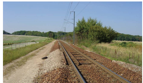
Figure 1. The concerned area of the railway track
