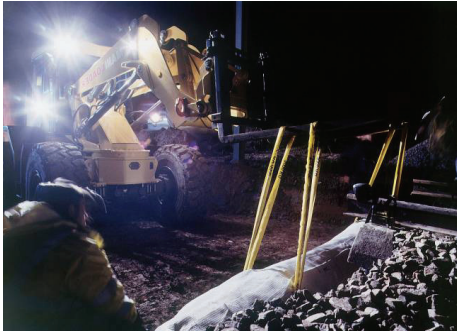
Figure 7. Installation of the roll during the night
