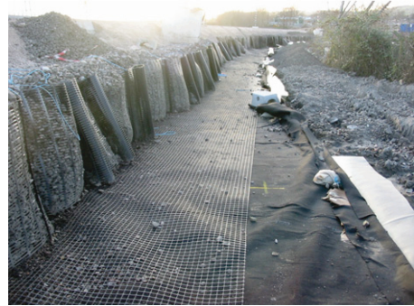
Figure 5 Detail of the geosynthetic capping.
