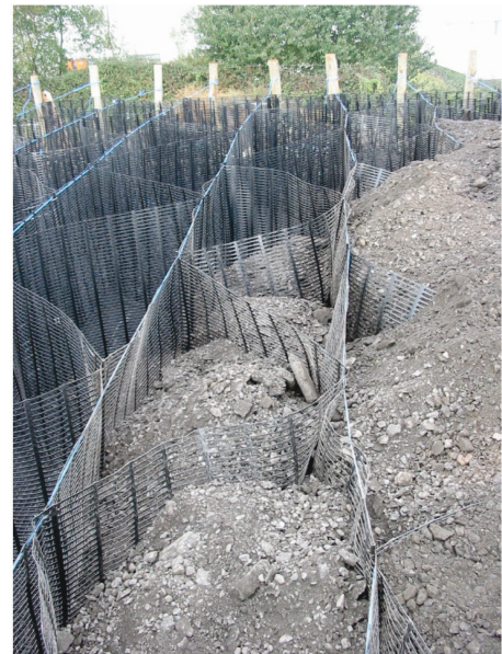
Figure 6. Geocell mattresses during construction.
