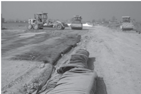
Figure 5. Both side anchorage of the cross resistant geogrid.
