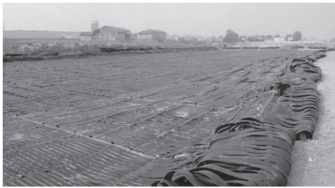
Figure 3. Installation layout of the cross resistant geogrids.
