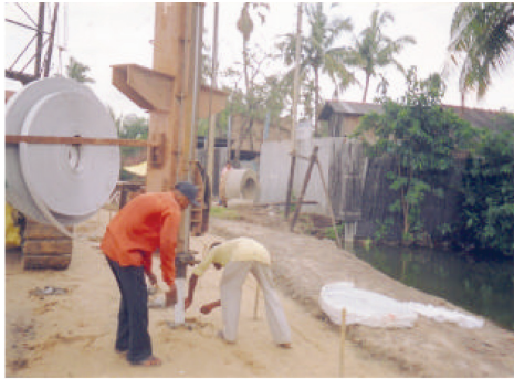
Photo 1. Installation of PVD.
