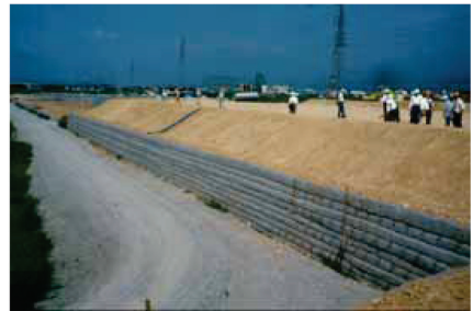
Figure 7. Completed pre-loading embankment.
