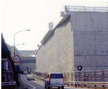
Figure 11. Completed wall with cantilever portion.
