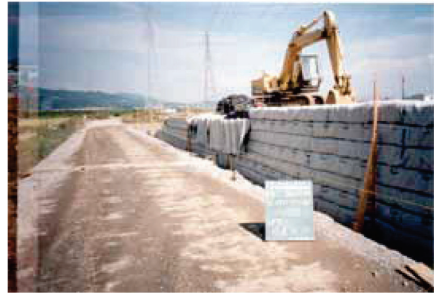
Figure 6. Construction stages of the embankment.
