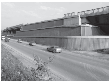
Figure 5. Completed south three-tier structure.
