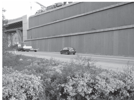
Figure 6. Completed north three-tier structure.
