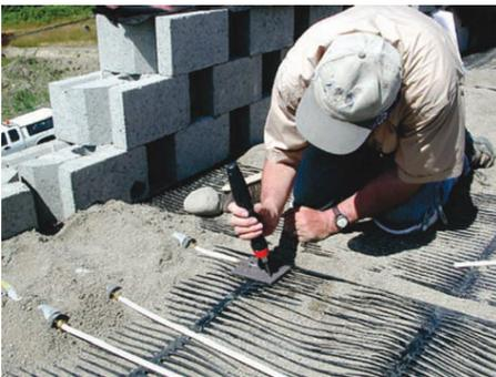
Figure 2. Installation of extensometers.
