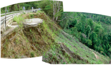
Figure 3. Failure of road at Km. 86+300 Hwy. 108.
