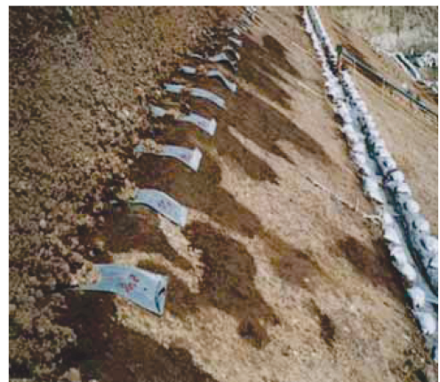
Photo 7. Drainage by geocomposites dark : wet by the drain water.
