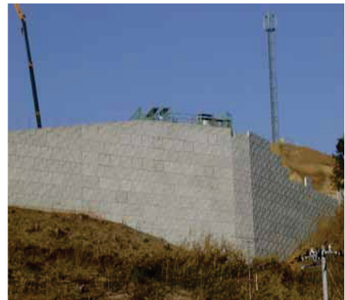
Photo 6. Reinforced walls with concrete facing unit.
