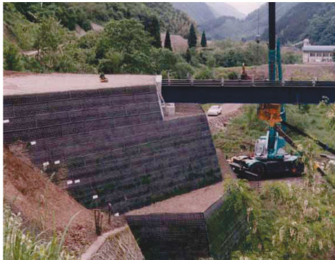
Photo 3. Reinforced wall abutment.
