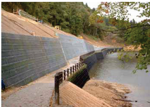
Photo 4. Reinforced wall along a walk road.
