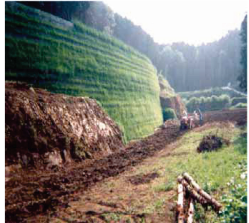
Photo 5. Reinforced wall road in mountainous area.
