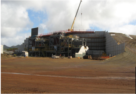
Figure 3. ROM Wall – close to completion
