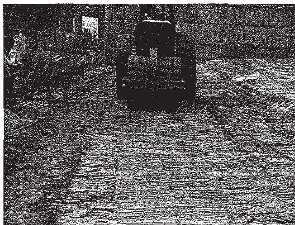
Fig. 3 Compaction of flyash
