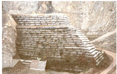
Figure 1. Testing slope with geogrid reinforcement.
