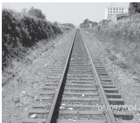
Figure 1. Railway crossing the city in East-West direction.
