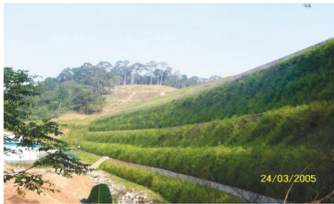
Figure 7. Completed Section of wall.
