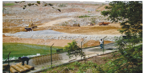
Figure 5. Rock-fill Base of Structure.
