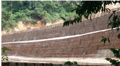
Figure 8. Panoramic view of wall.
