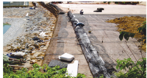
Figure 6. Base Layer of Woven Geotextile.
