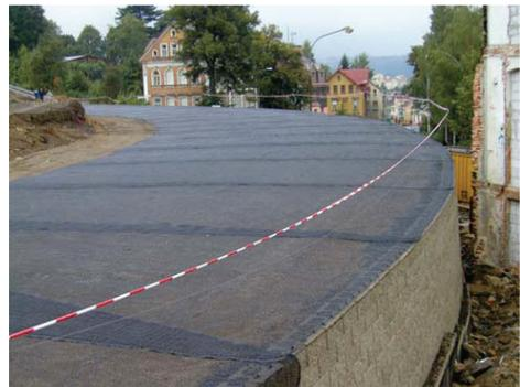
Figure 6. Jablonec, building reinforced soil structure near the house.
