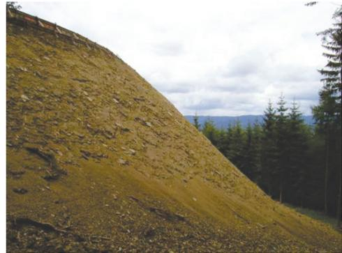
Figure 3. Vranca, 17 m high reinforced fill.
