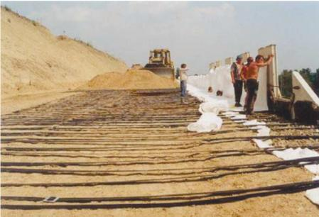
Figure 1. Mlcechvosty, spreading fill on strip reinforcement.
