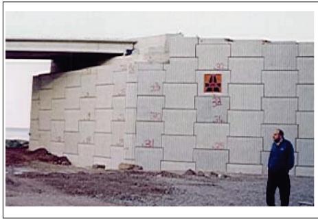
Figure 3. View of A2 abutment on K2A Junction.
