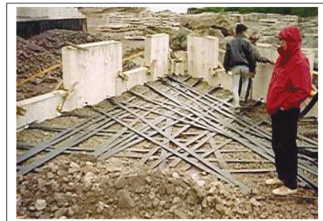
Figure 2. Polymer strip laying in A2 abutment on K2A Junction, Özçelik (2004).
