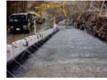
Photo-3 Situation of geogrid installation
