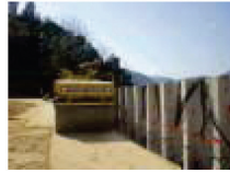
Photo-4 Situation of compaction adjacent to facing wall
