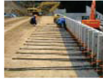
Photo-2 Situation of installation of anti-drawing material
