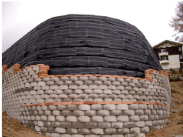
(a) Hybrid reinforcement (Before grass germination)
