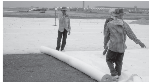
Figure 11. Laying of geotextile separator at New Bangkok International Airport Project, phase 2.
