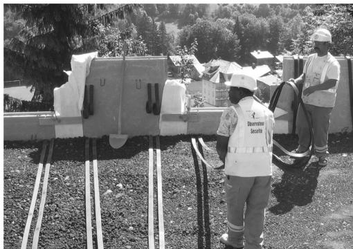
Figure 1. Construction of an MSE wall with geostraps.
