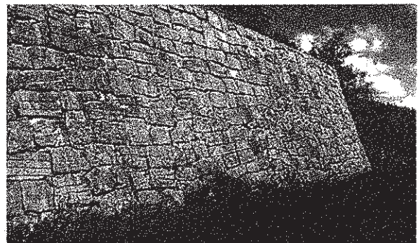
Figure 1. Polygonal masonry lining wall.
