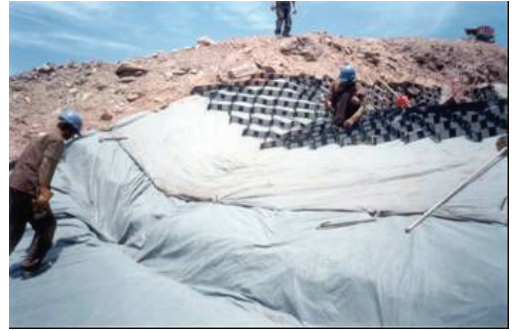
Figure 5. Opening the trenches and installing the geotextile.
