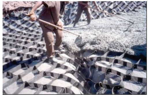
Figure 6. Infilling the geocells and the trenches with concrete.
