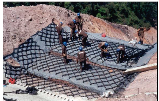
Figure 8. View of the intermediate berm.
