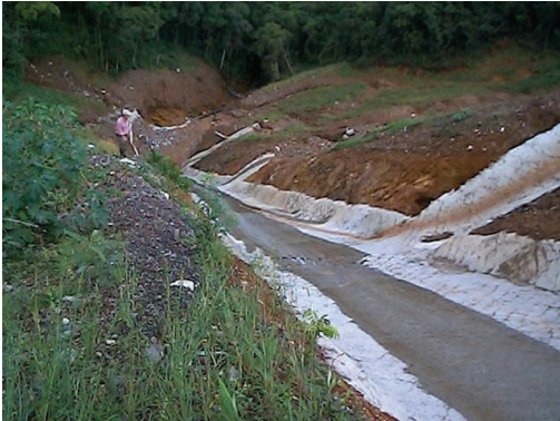
Figure 1: General view of channel.
