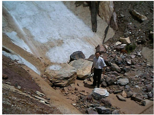
Figure 10. Stones deposited in the intermediate berm after intense precipitation.
