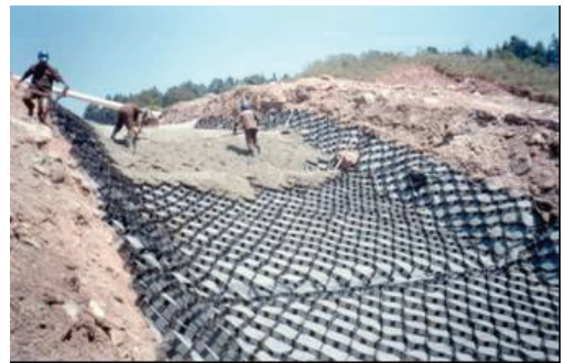
Figure 7. General view of the inclined portion of the channel.
