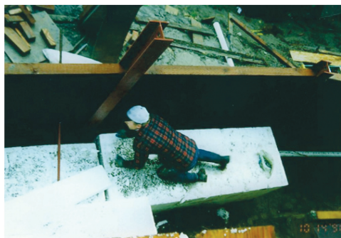
Figure 3. Geofoam block field installation.
