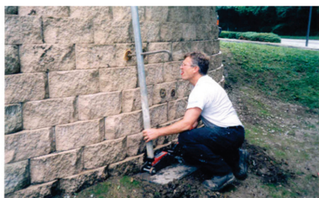
(c) Vertical pipe extending to auto jack
