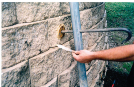
(b) Steel bar in lifting sleeve and through pipe
