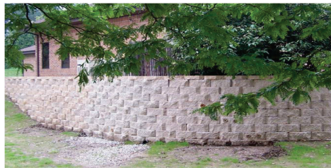
(b) Photograph of wall
