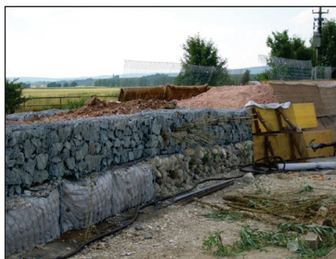
Figure 4. Inserting of willow branches.
