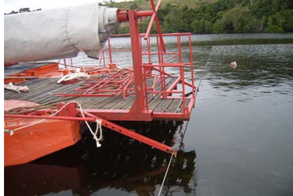
Figure 9. The cable used to guide the barge during laying operations
