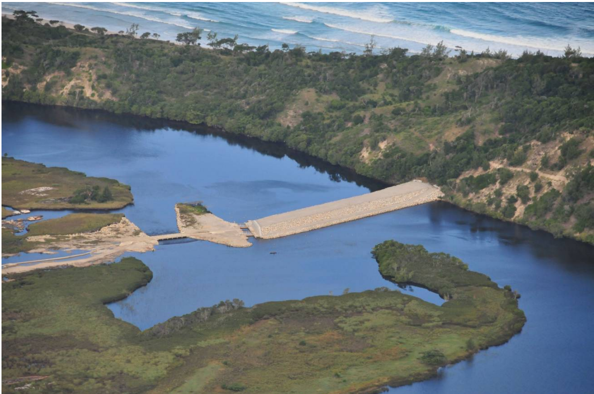
Figure 16. The completed embankment, boat lock and low flow spillway
