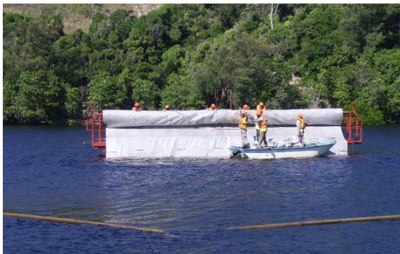
Figure 10. Laying the foundation geotextile layer from a specialised barge
