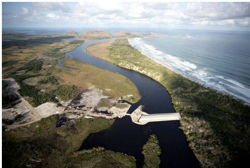
Figure 1. The Anony River Estuary and Partially Completed Weir
