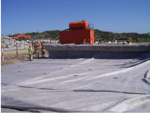
Figure 8. Preparing geotextile sheets prior to laying
