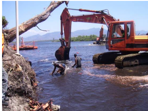
Figure 13. Closing the embankment against the right bank
