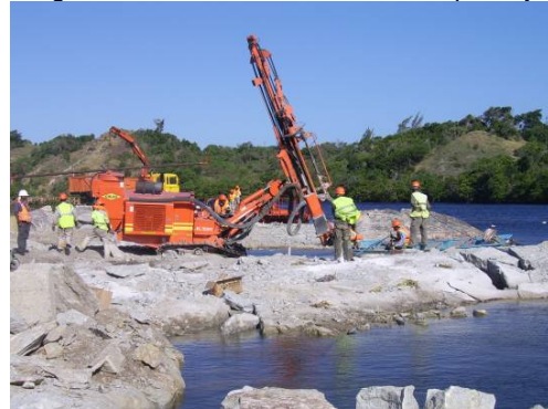
Figure 7. Excavation on the main spillway
