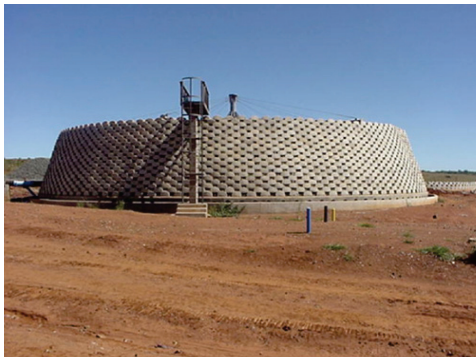
Figure 1. Concrete block trickling filter.
