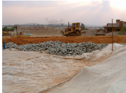
Figure 7. Preparation of final levels.
