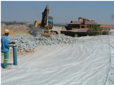
Figure 6. Placement of dump-rock.
