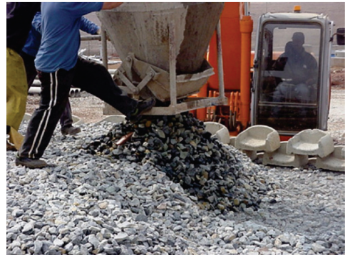
Figure 2. Placing of stone.
